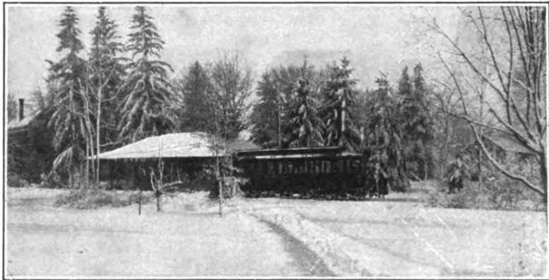
Cooperative Store and Trolley Depot.
